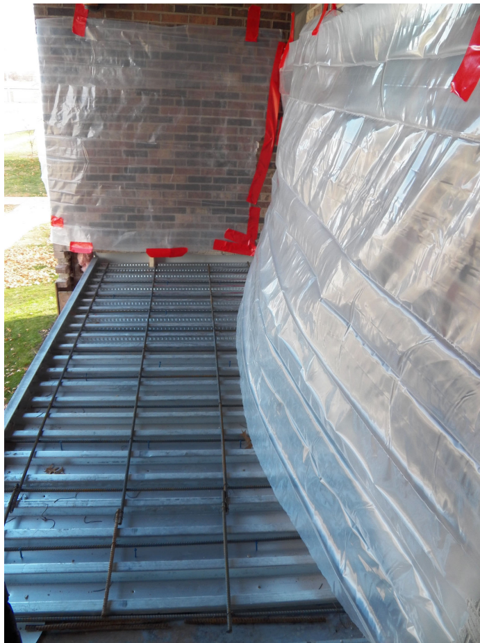
4. Reinforcing steel in place at Building A3.
