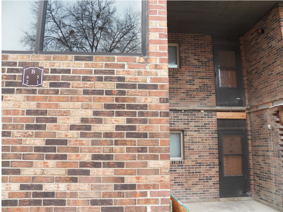
1. Balcony removed at Building A2.
