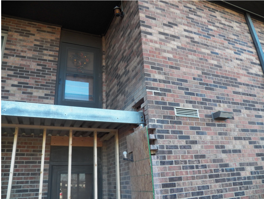
1. Steel set at Building A5.
