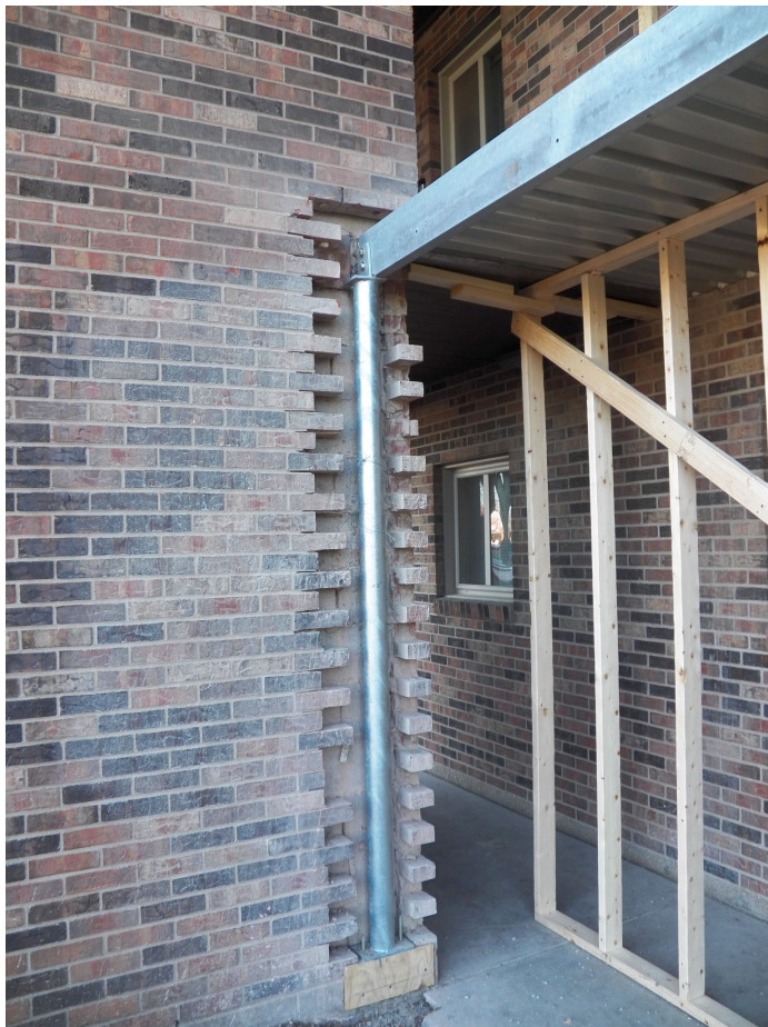
2. Steel set at Building A5.
