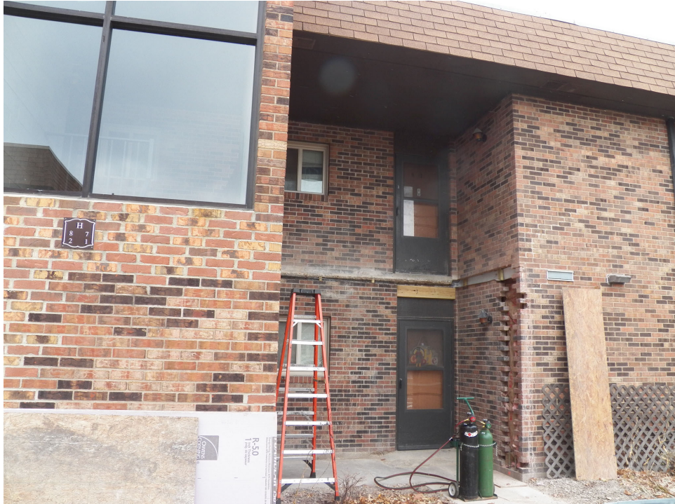
7. Balcony removed at Building B6.
