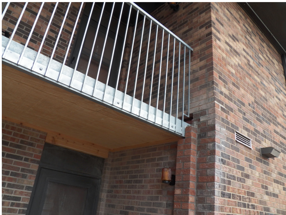
4. Brick pier at Building A5.
