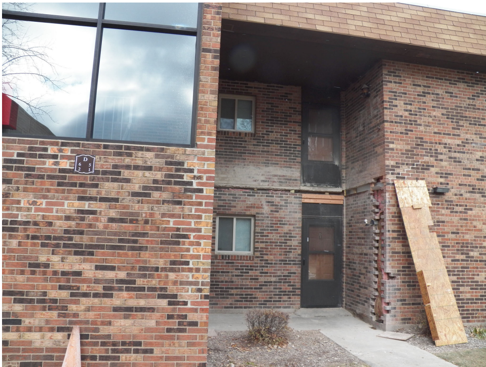
6. Balcony removed at Building A4.
