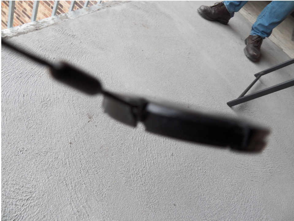
5. Floor texture good match at Building A5.
