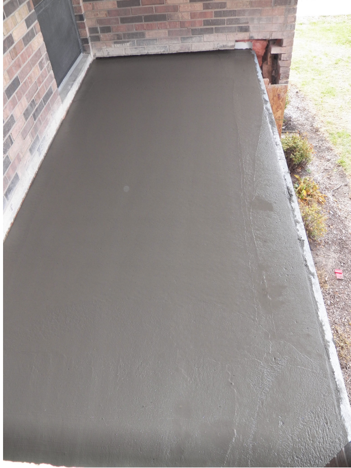
5. Concrete in place at Building A5.
