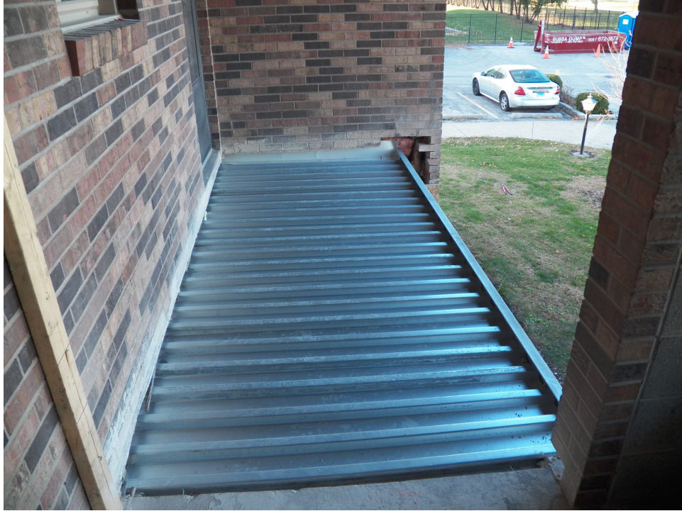
3. Forms in place at Building A5.
