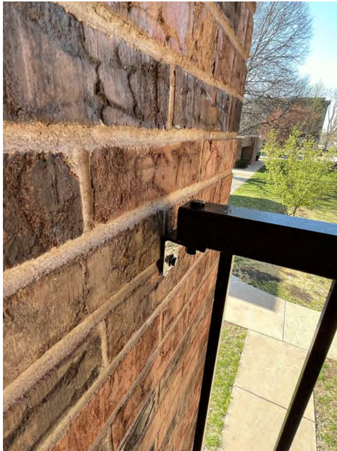
2. Thru-bolt fastener at railing/wall attachment (typical).
