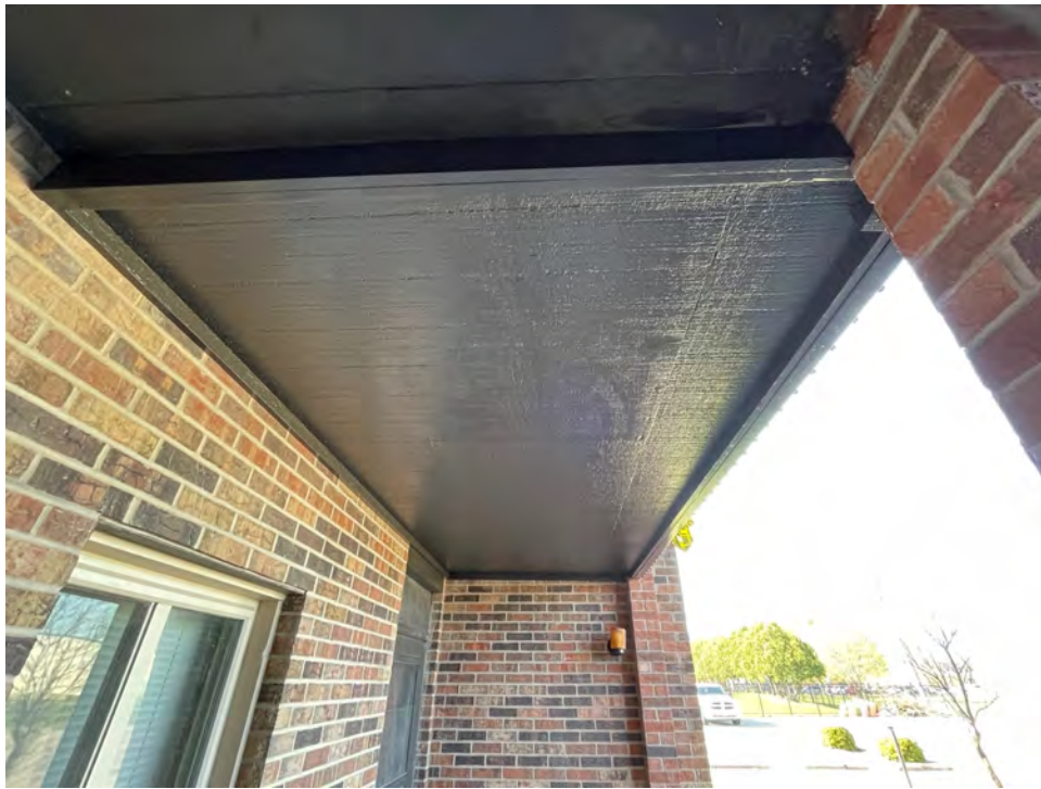
1. New painted plywood soffit (typical) at all replaced balconies.
