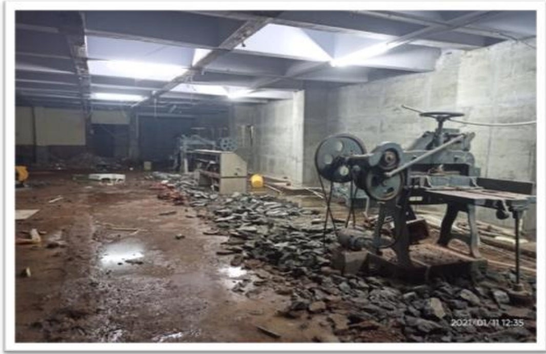
Archive facility – after completion of the refurbishment work
