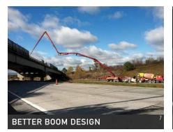
Robust and more resilient, Putzmeister's "smart design" boom incorporates welding seams below the edge of maximum stress. The boom is engineered to offer the flexibility to adapt to different loads and features more straight pipe for a less stressful concrete flow and longer wear on parts. The Z-Fold configuration handles space restrictive areas and can pump even if the boom is not fully extended.
