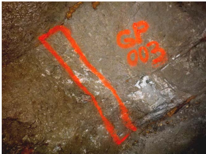
Picture 7.1. La Criolla vein on a mining drift, channel of 130 cm, level 595.
