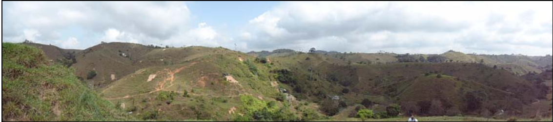
Picture 5.3.- Panoramic view of the Palmichala property. View south to north.
