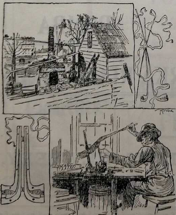
VIEW OF EXTERIOR AND INTERIOR OF CLAY PIPE FACTORY.
