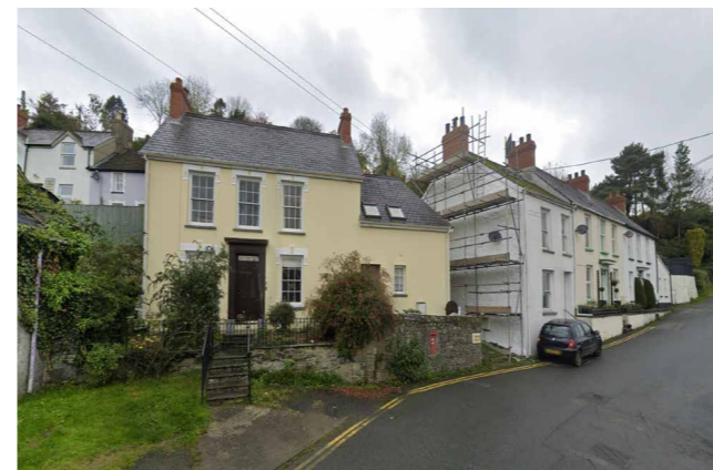
2 Storey house at the entrance of the street
