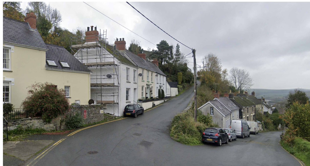
2 Storey units at the junction of Pen-Y-Rhiw and Tan-Y-Rhiw
