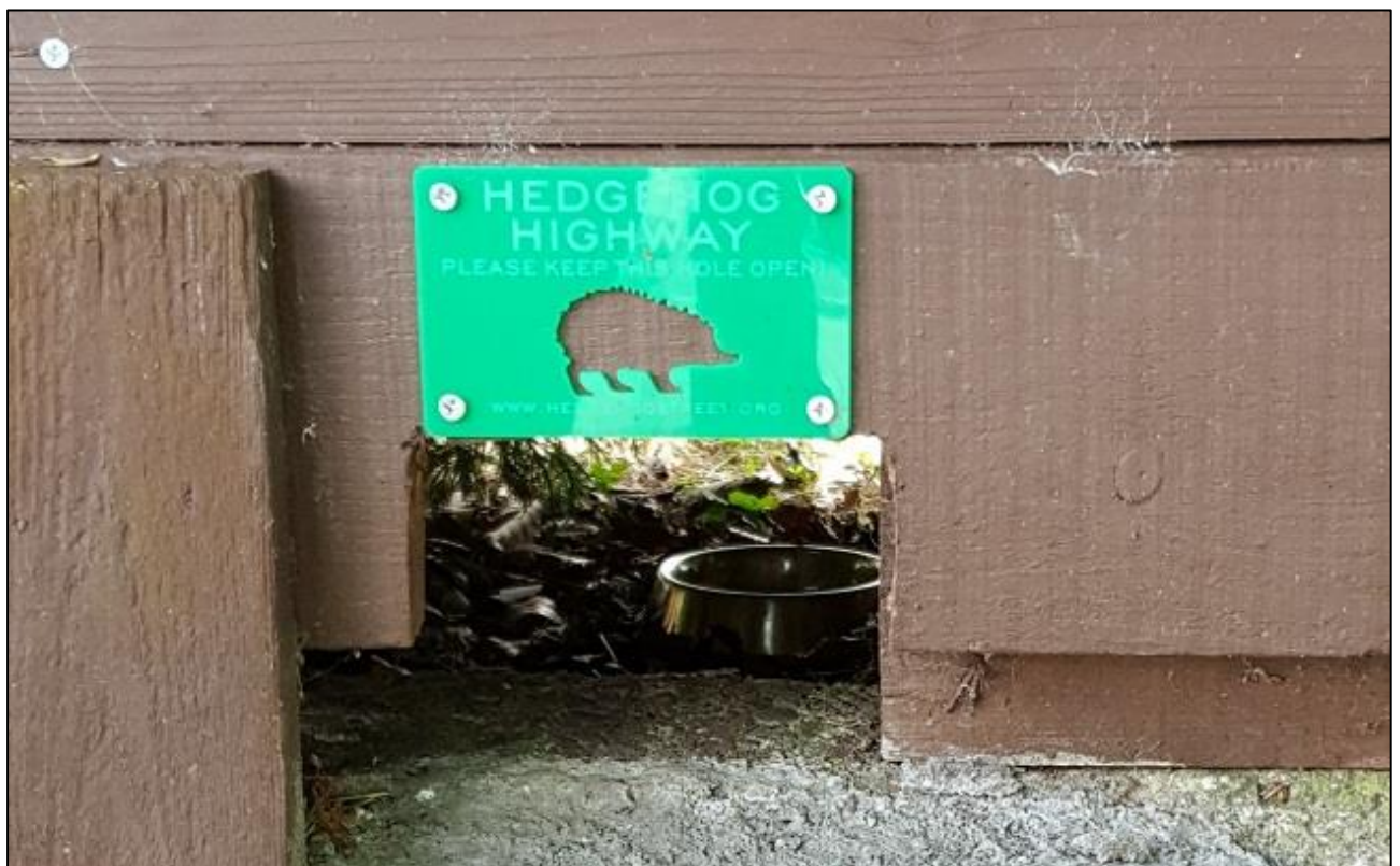
Figure 18. Hedgehog highway included in base of fence to allow hedgehog movement.
