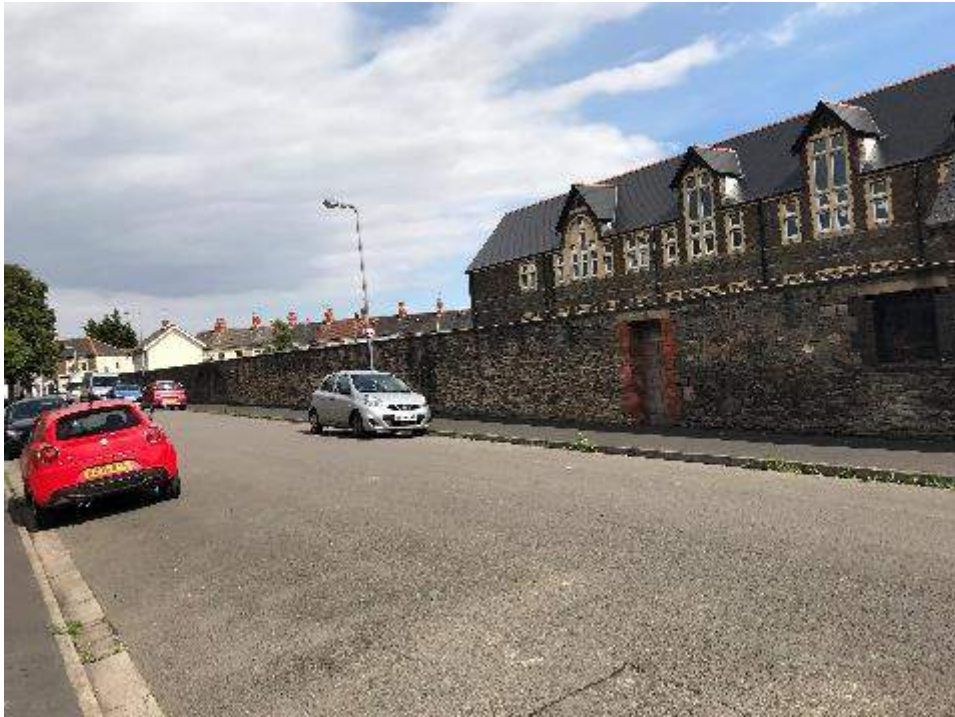
Photograph 42: View towards application site.
