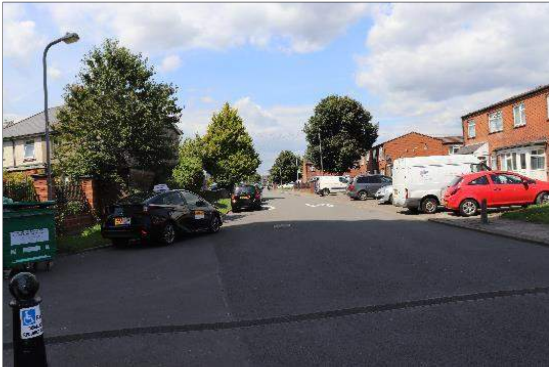
Photograph 13: Channel View Road through the centre of the application site, facing north.
