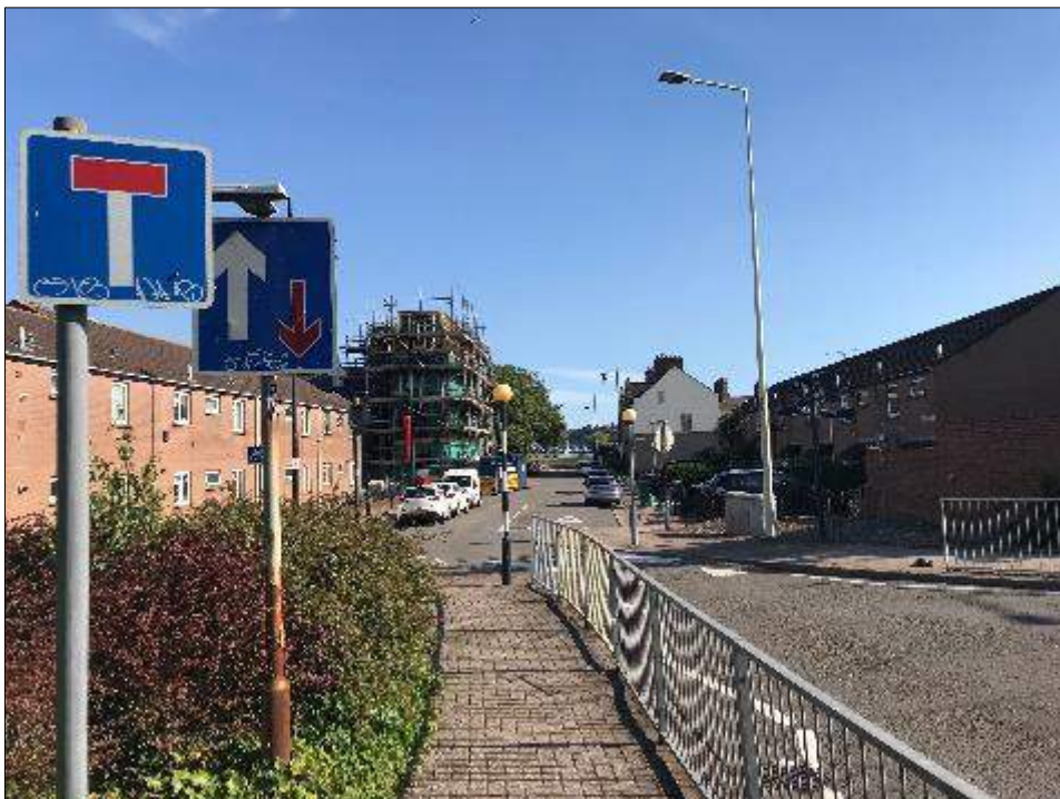
Photograph 58: View towards application site.
