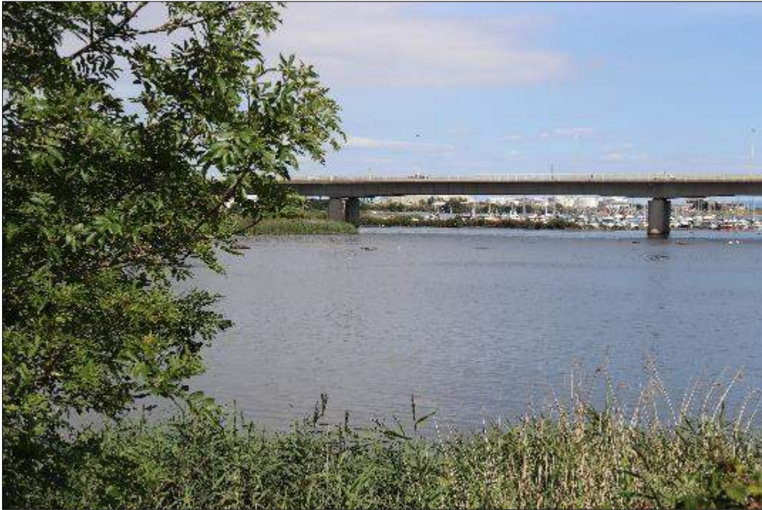
Photograph 24: View of GM553, facing east.
