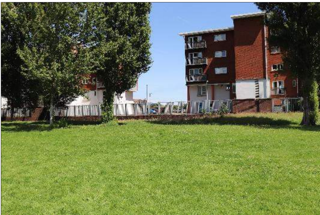
Photograph 6: North-east of the application site, facing Jim Driscoll Way, facing east.
