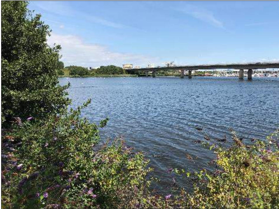
Photograph 28: View of GM553, facing north-east.
