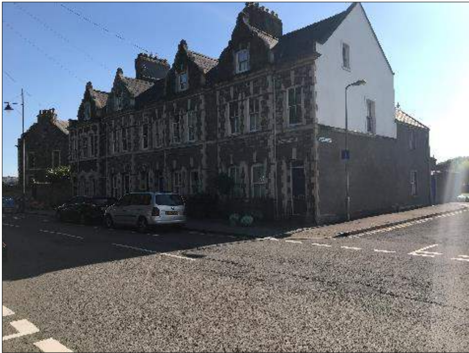
Photograph 55: View towards application site.
