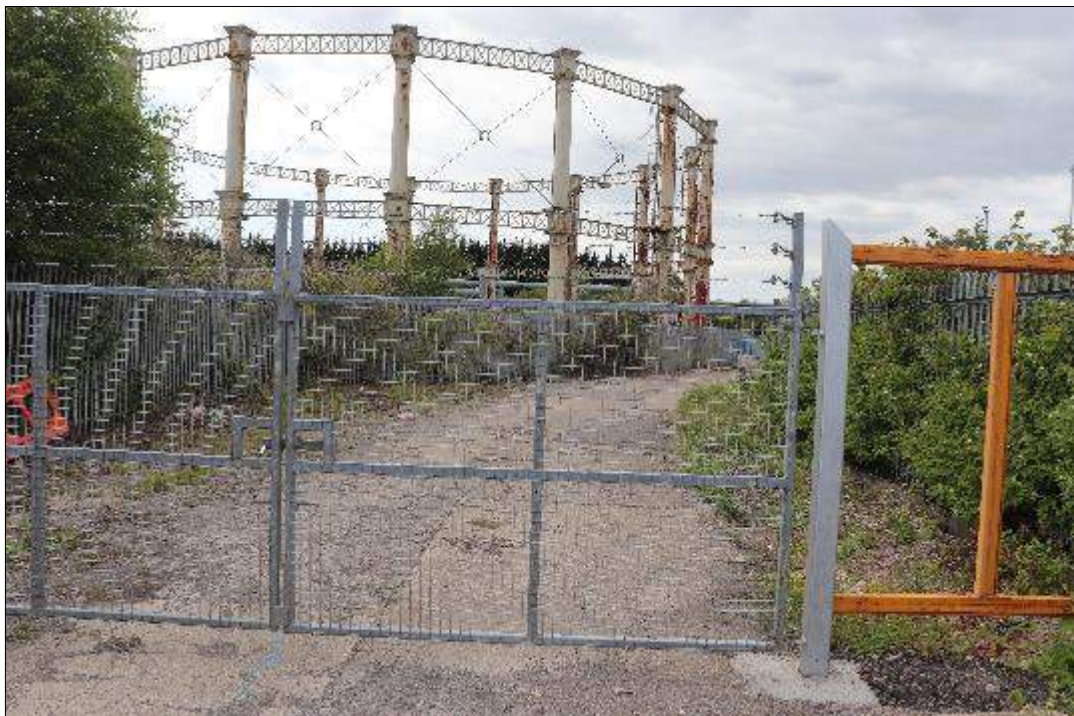
Photograph 37: View of Gas Holder.
