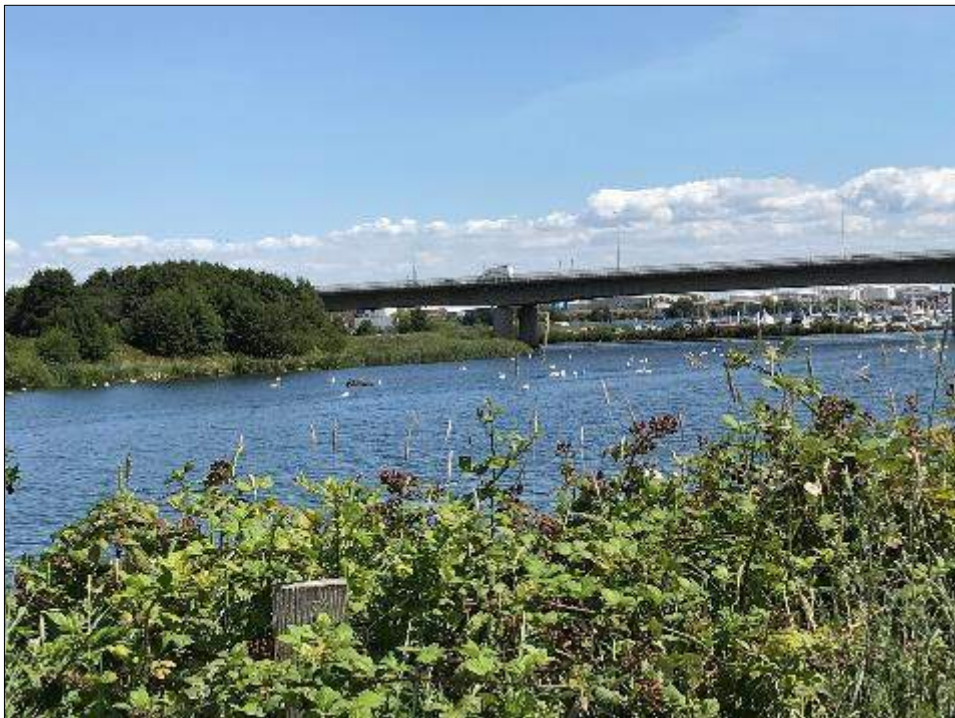
Photograph 27: View of GM553, facing east.
