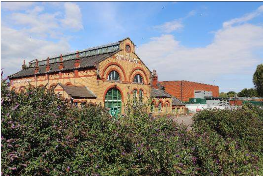
Photograph 35: View of Pumping Station, facing north-west.
