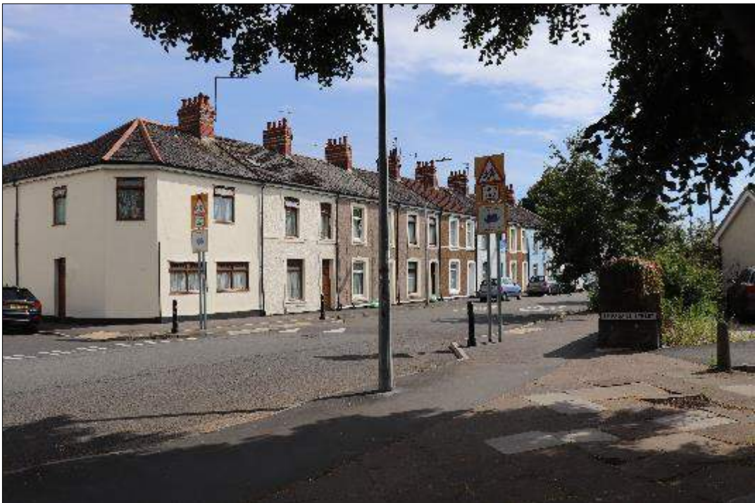
Photograph 45: View towards application site.
