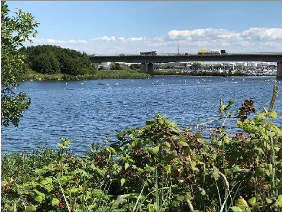
Photograph 26: View of GM553, facing east.
