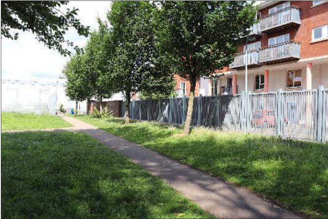
Photograph 8: View of north-east of the application site.
