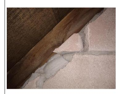
Water ingress. Plaster has failed.
