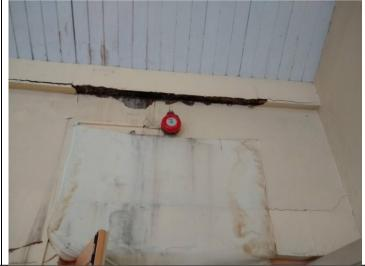
Window does not shut fully. Very narrow (2mm) gaps around frame. Wire mesh on outside but gaps large enough for bats to enter.
