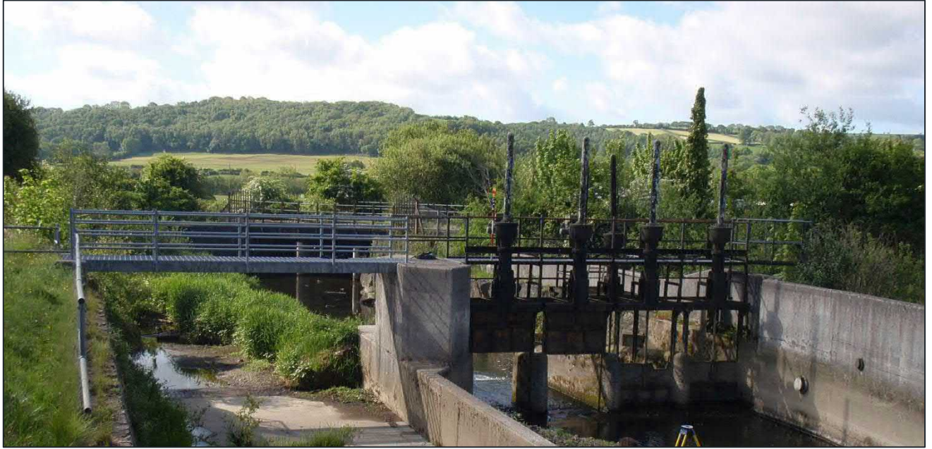
Figure 1-4: Site sluice structure (showing overflow channel, left bank) 5
