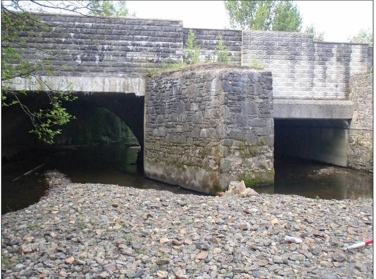
Figure 1-2: Market Street Bridge 3
