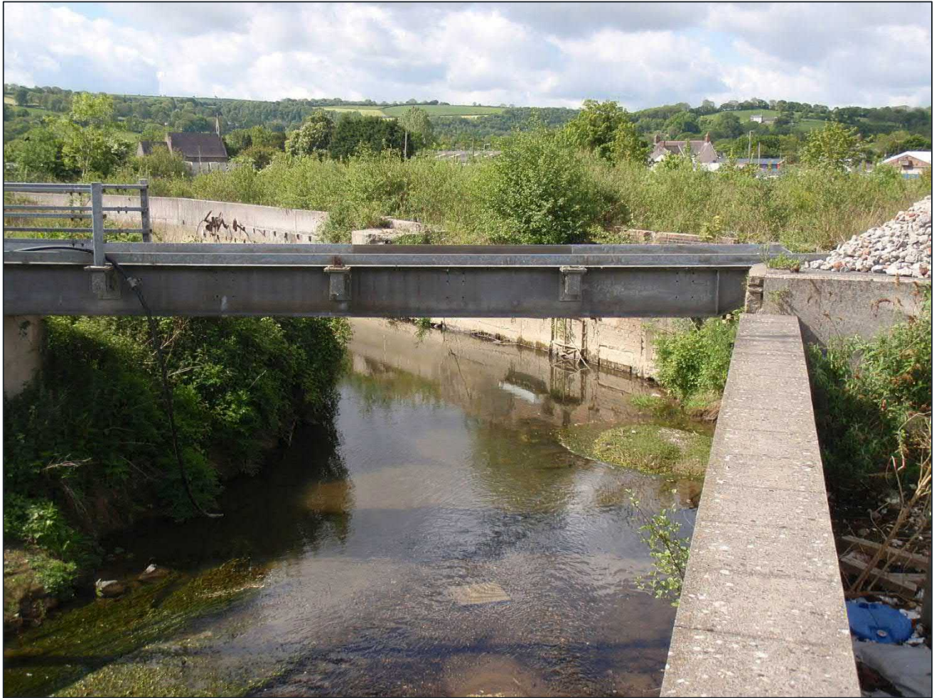
Figure 1-3: Site Footbridge (showing defence wall, right bank) 4
