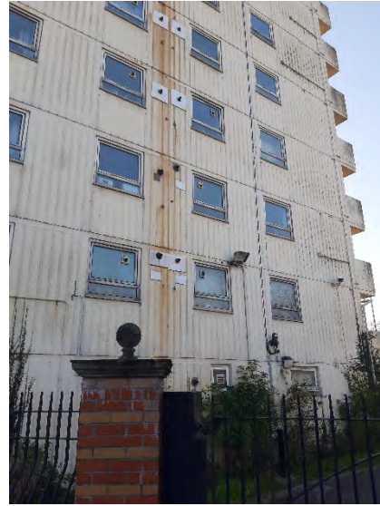
Plate 7- Channel View Road high rise flats cladding
