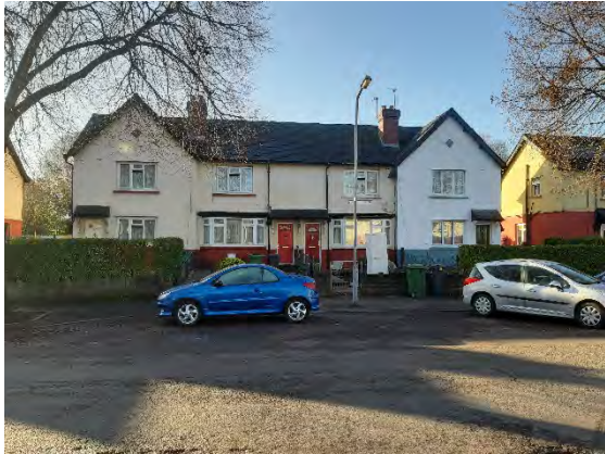
Plate 1- 50 to 64 South Clive Street
