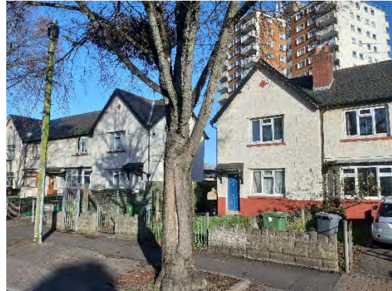
Plate 2- 117 to 127 South Clive Street
