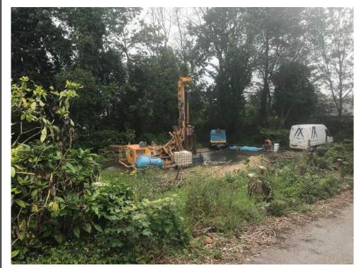
Plate 17: View of the KLEMM Rotary borehole rig, in position on BH01.
