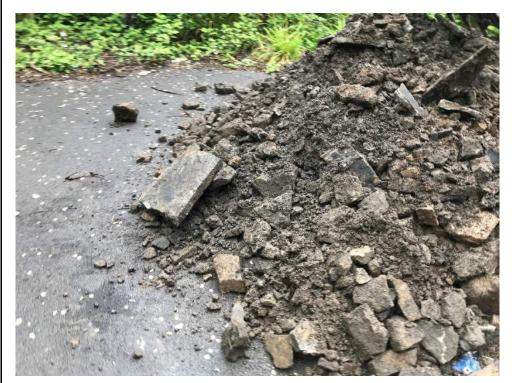
Plate 13: TP206 Spoil after excavation, displaying the Weathered Grovesend Formation bedrock encountered.
