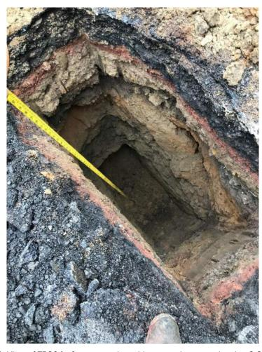
**Plate 10:** View of TP204 after excavation with measuring tape showing 3.3m depth.
