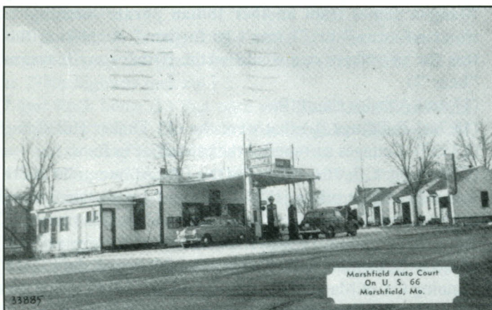
MARSHFIELD AUTO COURT. Begun by H.P. Highfill as a Shell station (1930), by 1947 (this postcard) Edward Petersdorf & Son were selling Standard "gas, cold drinks, and lunches," and renting the four cabins with garages.
