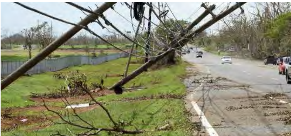
Infrastructure damage in Puerto Rico
