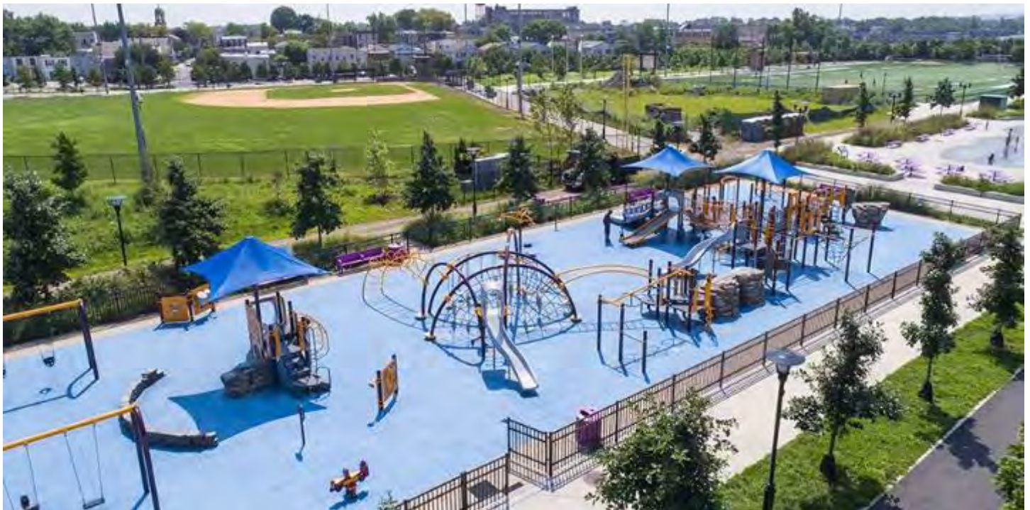
Before (above) and after cleanup and redevelopment of the Berry Land Park in Jersey City, New Jersey.
