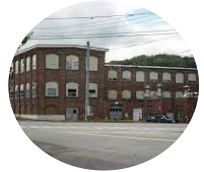
Village of Oriskany: Waterbury Felt Restoration $2M
