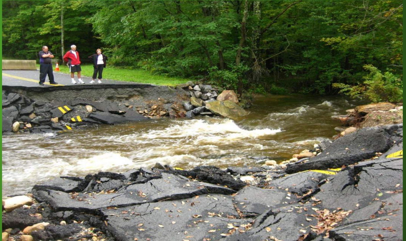
Bonny Hill Rigg Road, Becket Stream Crossing (TS Irene)
