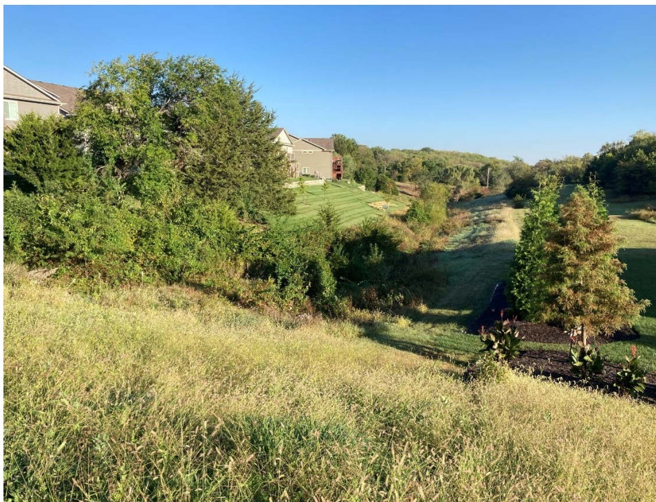
Figure 6 - View from the retention pond embankment looking north along drainage channel
