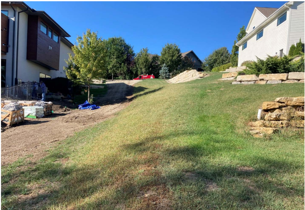
Figure 11 - 18% grade at Tract "A" connection to Landon Court.
