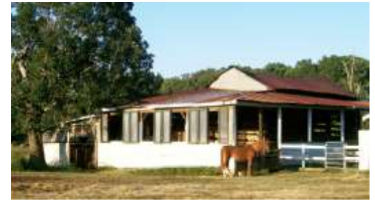
The west side of the barn repaired.
