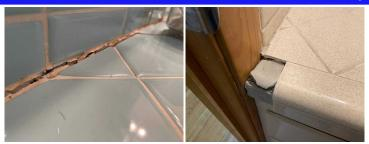
19. Bathroom Tub: Sealant at the base of tub in master bathroom is worn, cracked or missing. Recommend sealant.
