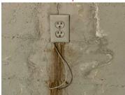
8. Moisture Present: Moisture at the east wall present at the time of inspection. Future evaluation and repair by a qualified basement waterproofing contractor is recommended.
