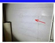
25. Movement: Past structural movement is suspected. There are multiple exterior cracks, interior wall/ceiling cracks, and foundation cracks. Further evaluation by a qualified foundation contractor is recommended.
