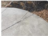
2. Patio: Paver, Concrete - Cracks and settling noted. Consider repair.
