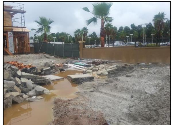
Poor stockpile management is demonstrated above. Rubble piles of asphalt and concrete were not covered and bermed before a rain event.
