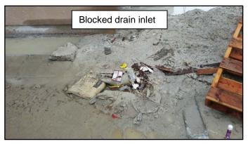
Upstream drains that have been compromised lead to increased run-on to the construction site. Run-on results from flooding when drains are compromised. It is not always the responsibility of the site to monitor all surrounding drains; however, it will benefit you if adjacent drains are inspected and cleared when a storm is forecasted to occur. Document any potential problems and report them if necessary.
