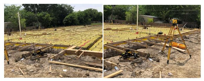
The foundation has been formed up and was being double checked for level before the concrete was poured.
