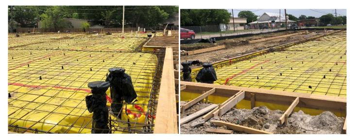
The Poly barrier and steel reinforcement has been installed. Plumbing pipes have been wrapped with poly prior to pour.
