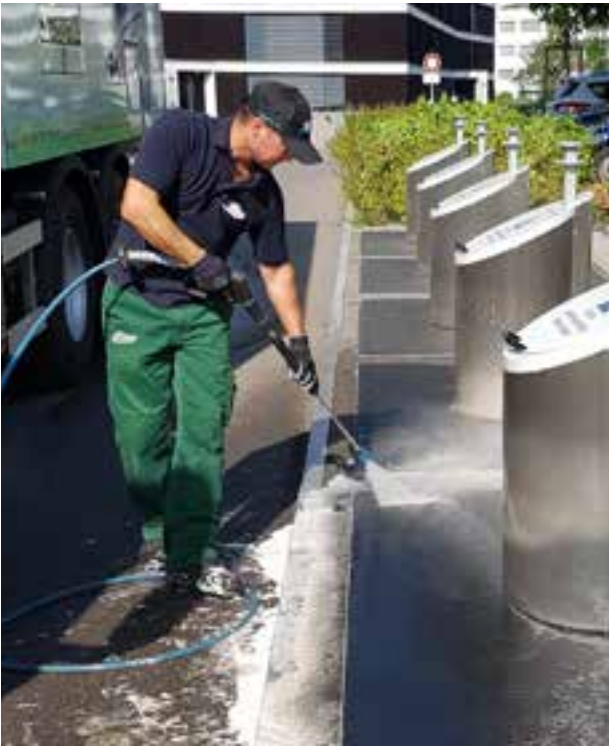
All residual soiling is removed with high-pressure and pre-spray cleaners.
