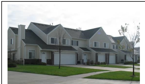
Example of Single-Family Attached
