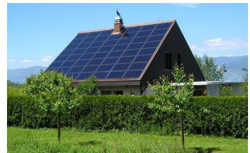
Example of a Solar Conversion System, Structure-mounted
