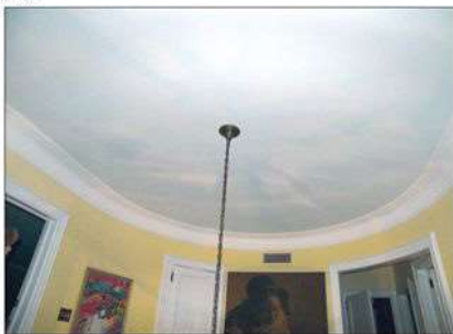
PHOTOS COURTESY CREATIONS IN PLASTER
