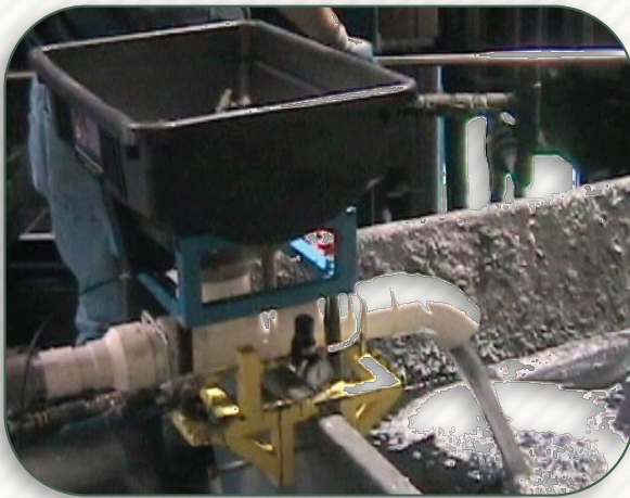
Latex flowing through feeder mounted to dump cart
