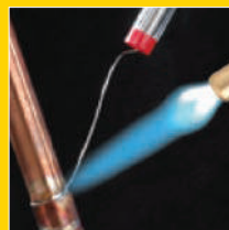
Soft Soldering
