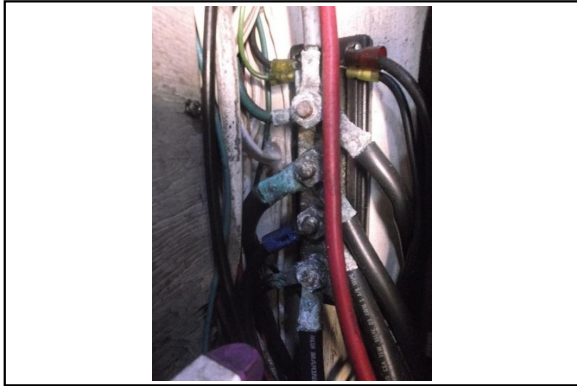
Terminal Corrosion
