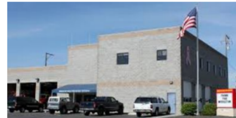
STATION 53 302 E. Main St., Middleton, ID 83644
