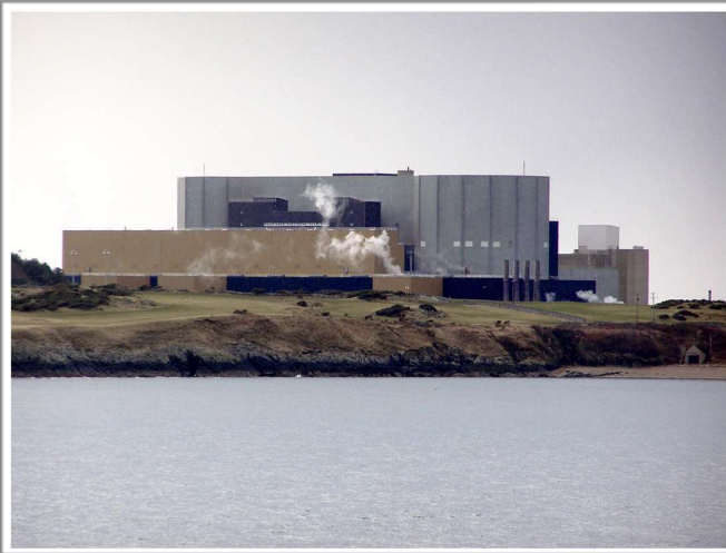
Wylfa Site. Photo Courtesy of David Dixon
