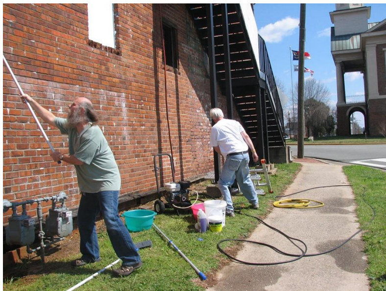
Scotty Young and Geo DeSocio power cleaning the mural wall
