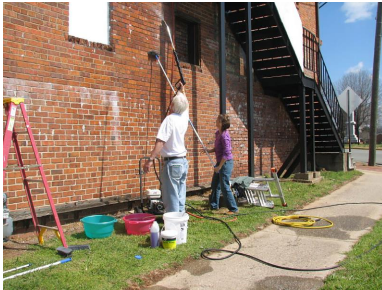
Diane and Geo DeSocio cleaning the Blair Building wall
