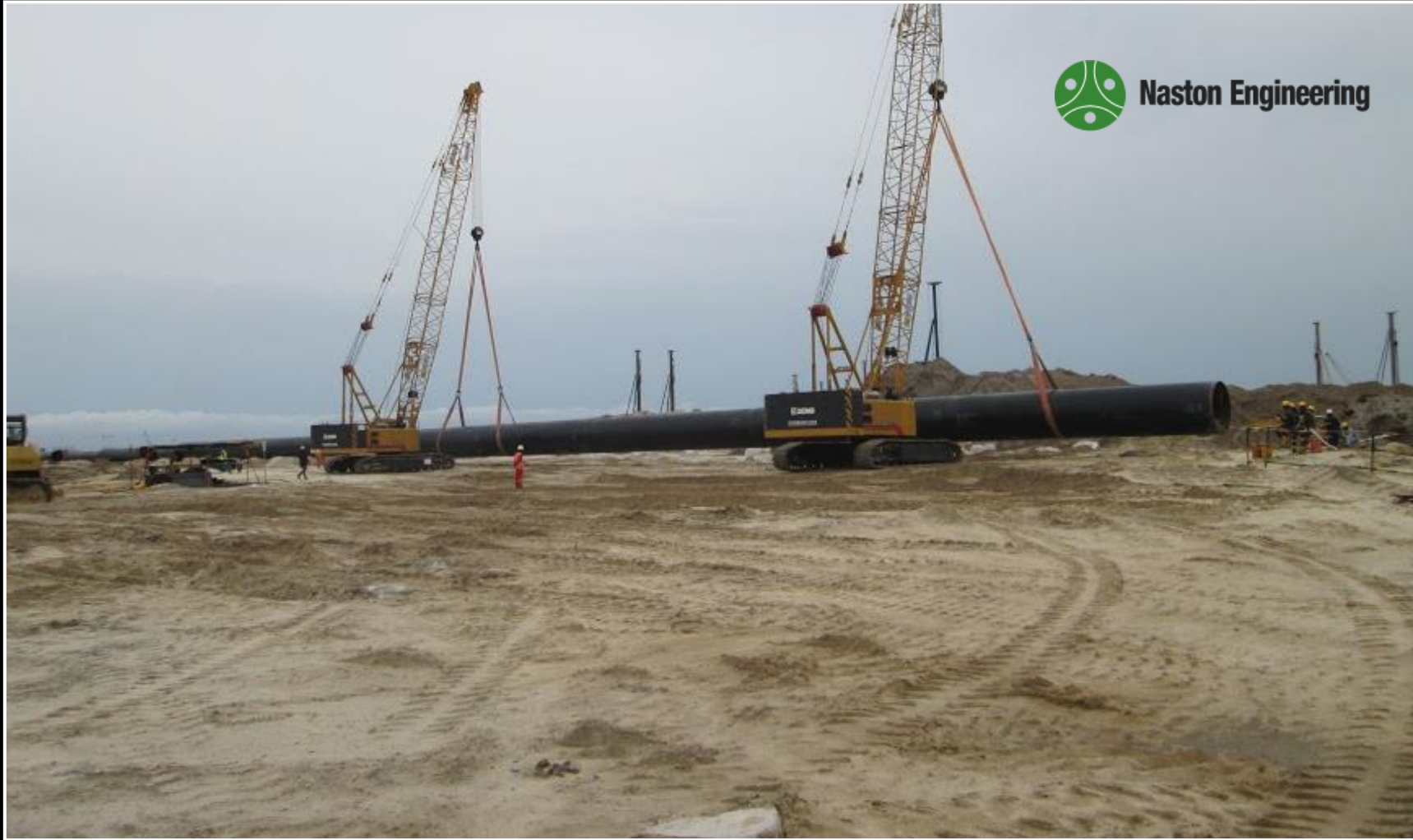
84" Pipeline Installation
