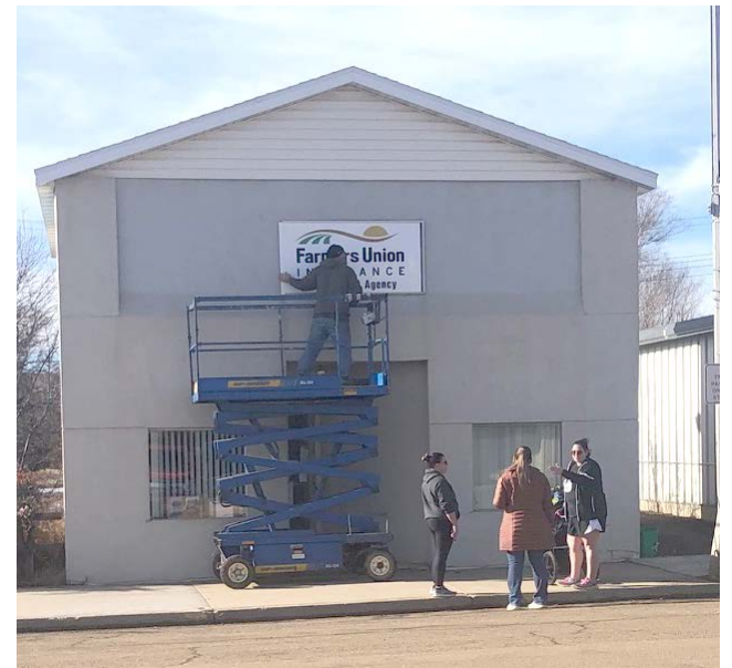
Kelly puts up new sign
