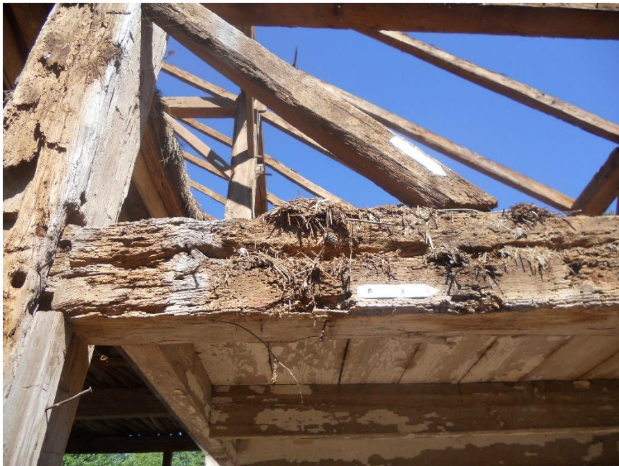
Massive crossbeams span the wide center aisle.
