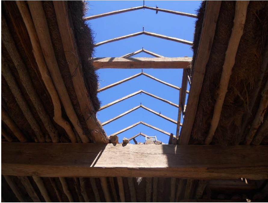
The steeply pitched gabled roof is visible through the hayloft
