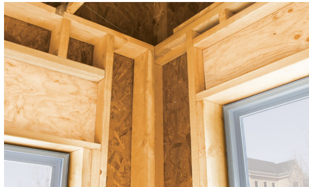
Insulated corners and headers are required for use of section 4.4.5 of the ENERGY STAR Thermal Enclosure System Rater Checklist. Two-stud corners (Figure 4) and single-ply headers (Figure 7) can be easily insulated to meet these requirements.
