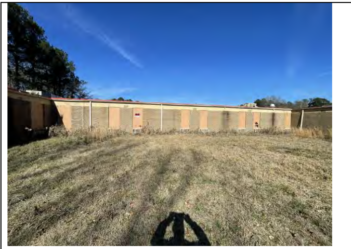
39. Window Frame Caulking and Windowpane Glazing
