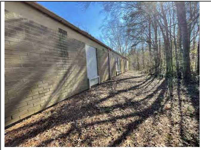
37. Window Frame Caulking and Windowpane Glazing
