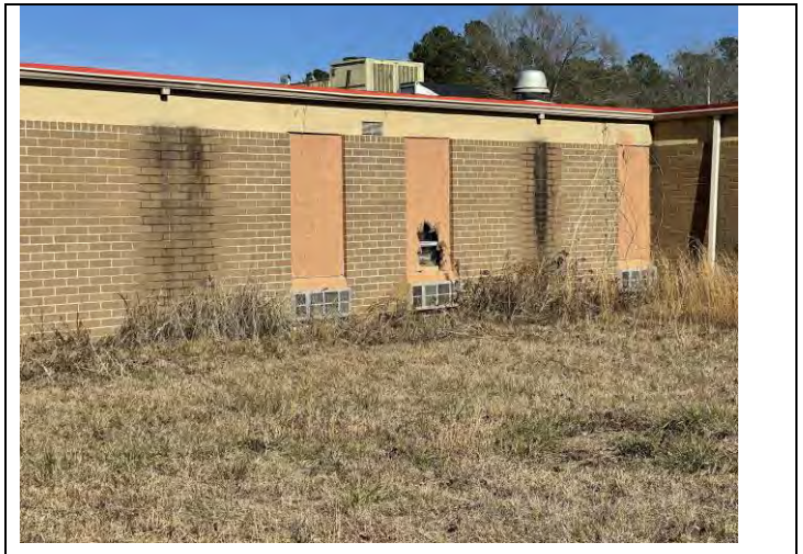
38. Window Frame Caulking and Windowpane Glazing
