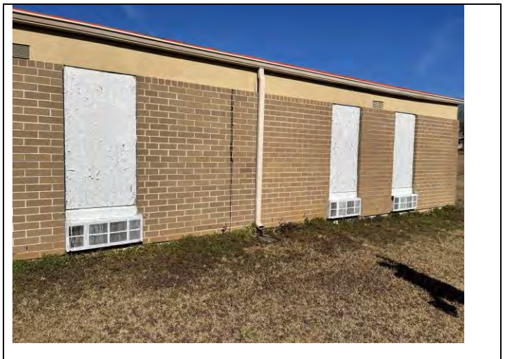
42. Window Frame Caulking and Windowpane Glazing
