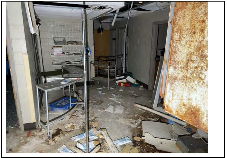
26. Pipe Fitting Insulation (Intact and debris on floor)
