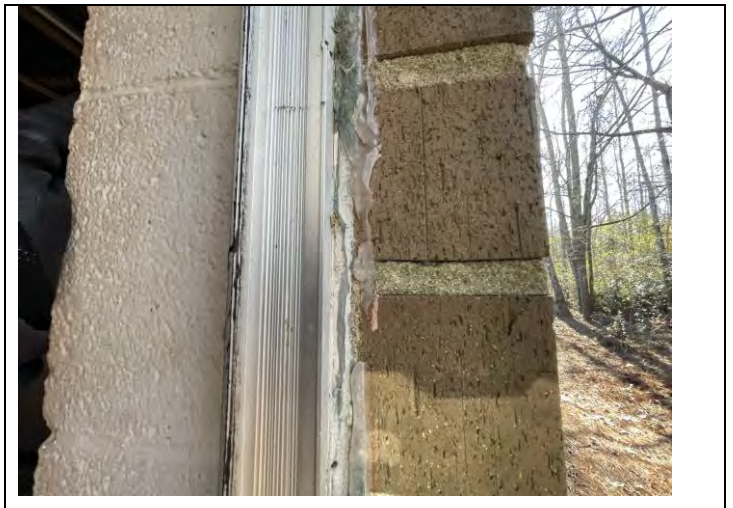
32. Window Frame Caulking and Windowpane Glazing
