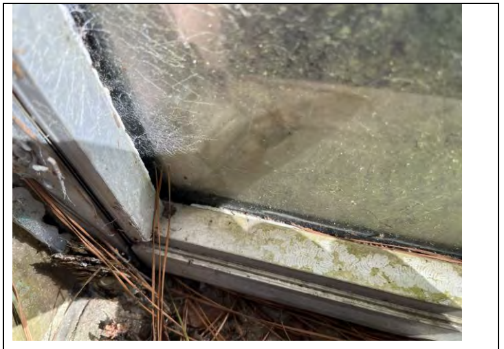
36. Window Frame Caulking and Windowpane Glazing
