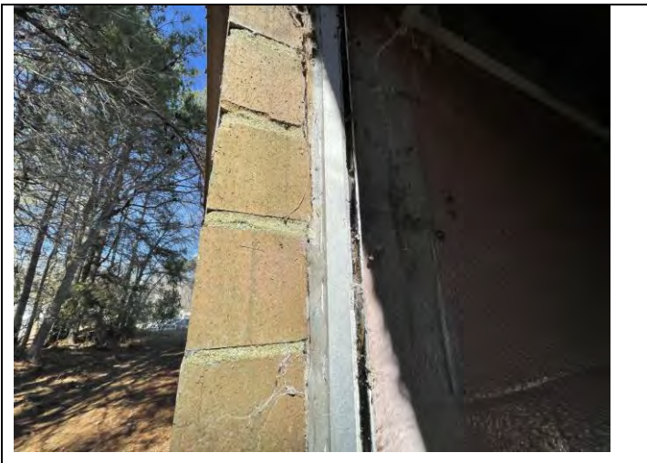
31. Window Frame Caulking and Windowpane Glazing
