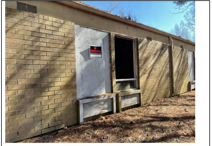
34. Window Frame Caulking and Windowpane Glazing
