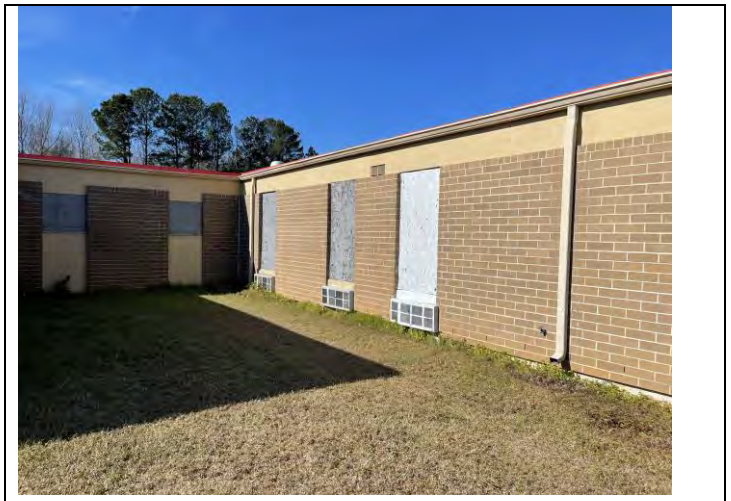
40. Window Frame Caulking and Windowpane Glazing
