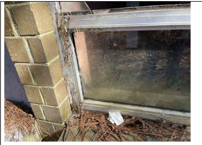
35. Window Frame Caulking and Windowpane Glazing
