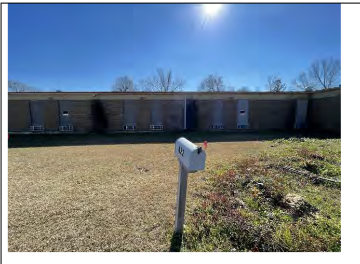
41. Window Frame Caulking and Windowpane Glazing
