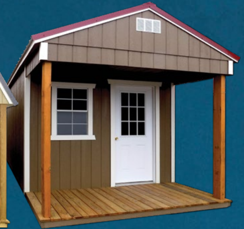
BROWN PAINT & BARN WHITE TRIM PAINT ON LP SMART PANEL SIDING
