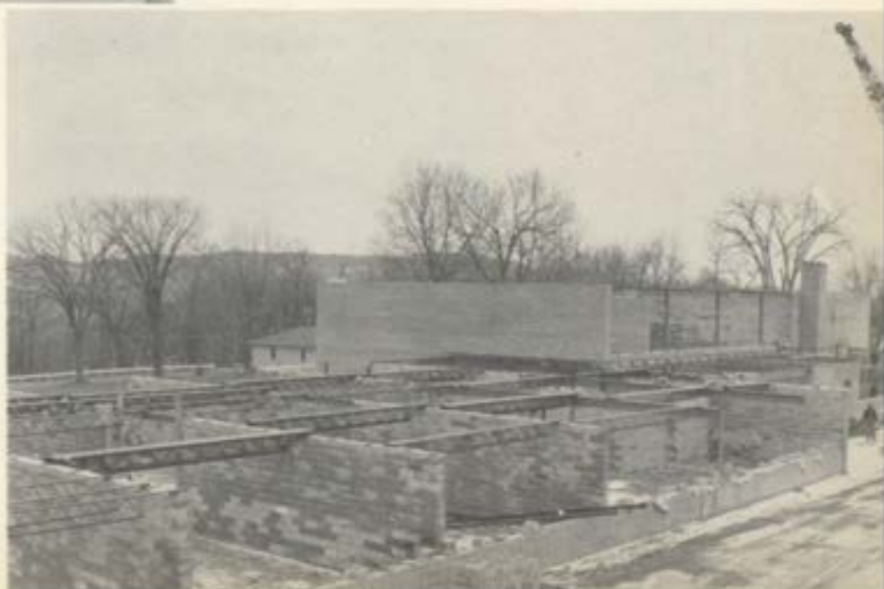
By January our new school is rapidly nearing completion.
