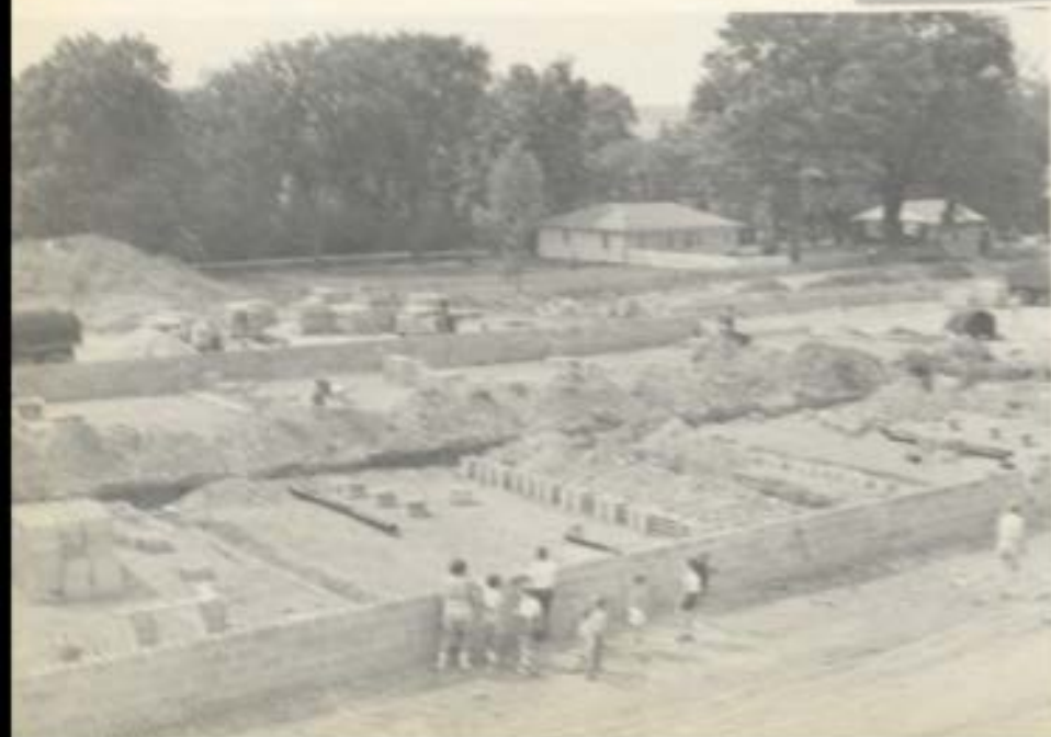
By August capable workers had completed the foundation of the building.
