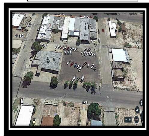
City Hall Parking Lot
