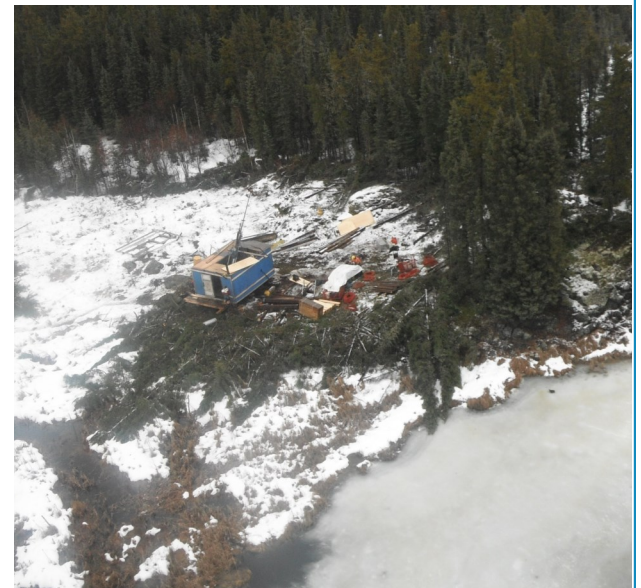
Drill Rig on Zoro Property
