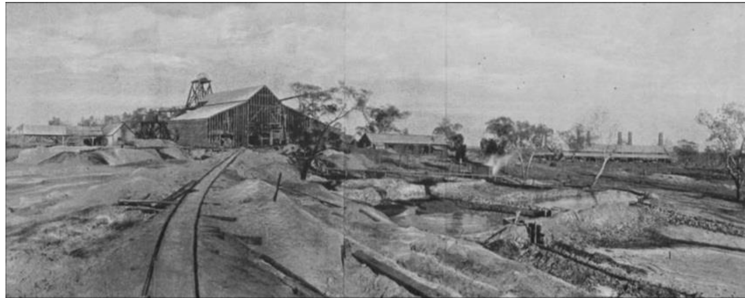
Girilambone Copper Mine, concentration, smelting plant and headframe (Carne, 1898) (Source: Coolabah Metals Ltd Prospectus, April 2022)
