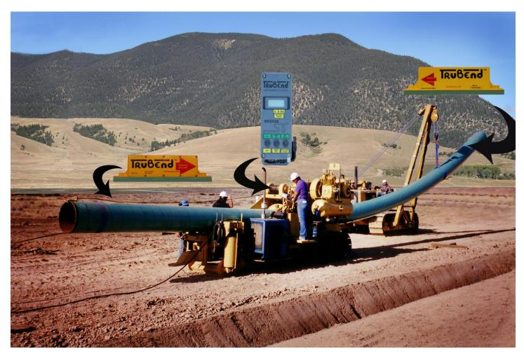
Mount the Receiver at the operators stand. Connect the power cable to the Bending Machine battery, black or brown wire negative and red wire positive.
