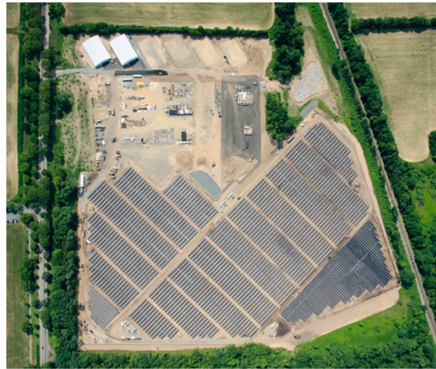
Princeton's Solar Panel Array
