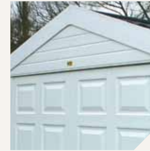
White PVCu fascias and vergeboards
