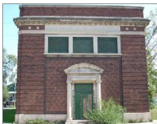
931 W. 120th Street (Fire Department Engine House)
