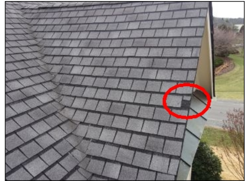
Damaged Shingles
