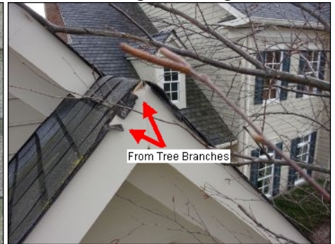
Damaged Shingles
