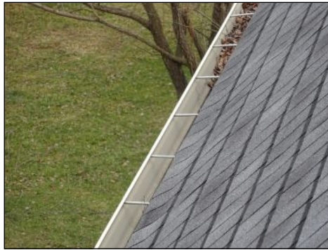
Partially Clogged Gutters
