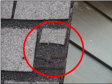
Damaged Shingles
