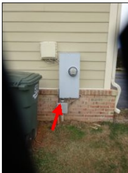
Underground Service to Meter
