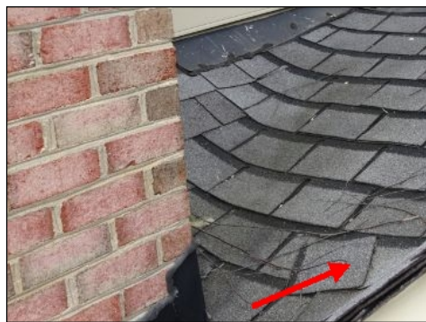
Damaged Shingles
