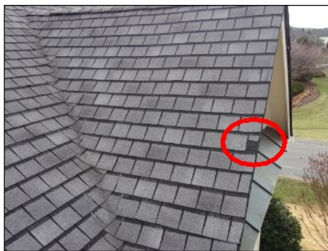
Damaged Shingles
