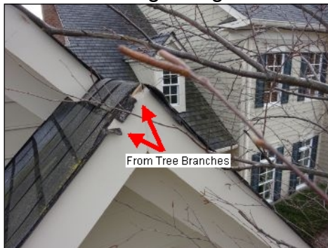
Damaged Shingles
