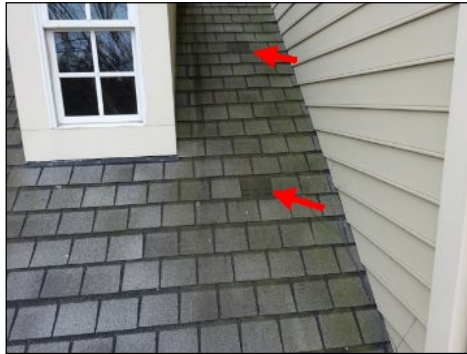
Missing Shingles
