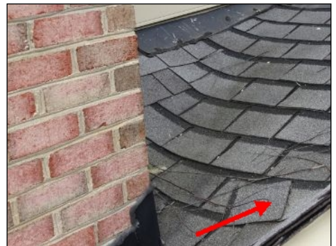
Damaged Shingles
