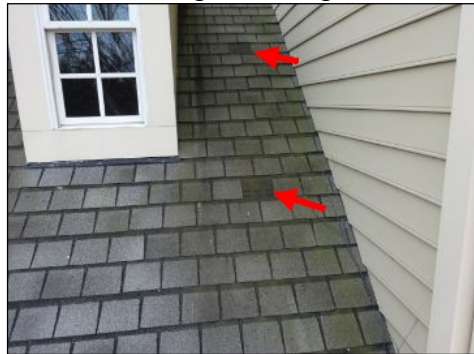
Missing Shingles
