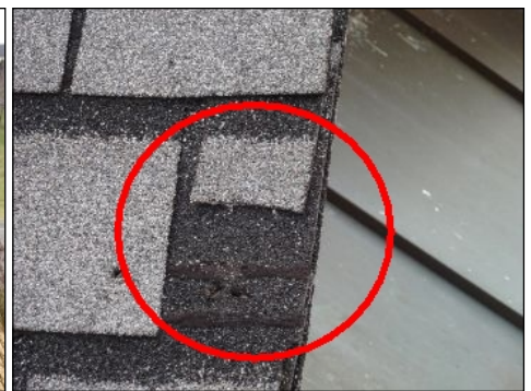
Damaged Shingles
