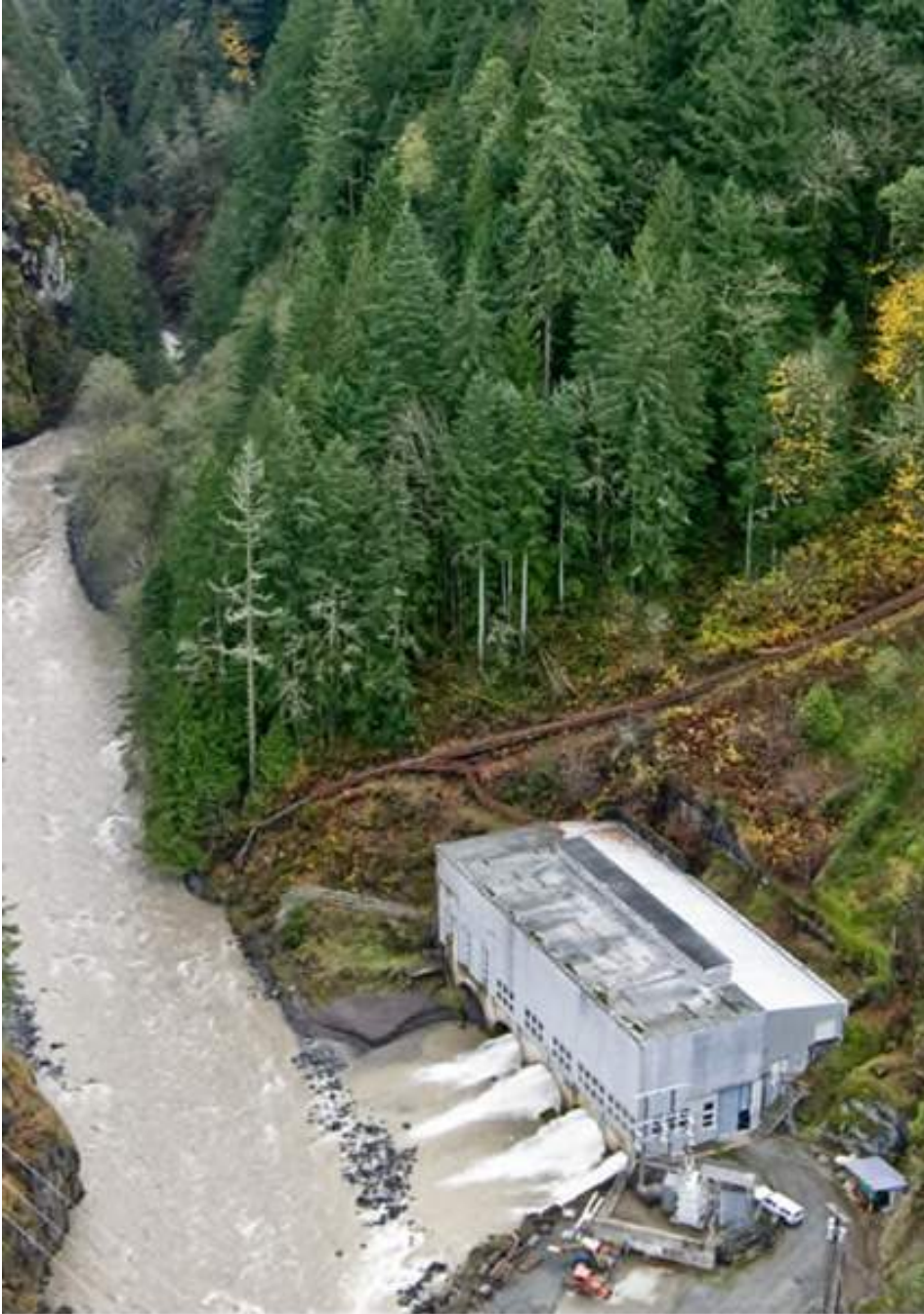
Figure _. Electron Powerhouse at RM 31.2
