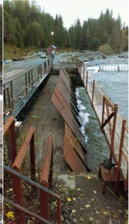
Existing Intake Wall & Flow Plates
