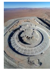
Foundation for the Extremely large telescope 39.3 meters when complete.
