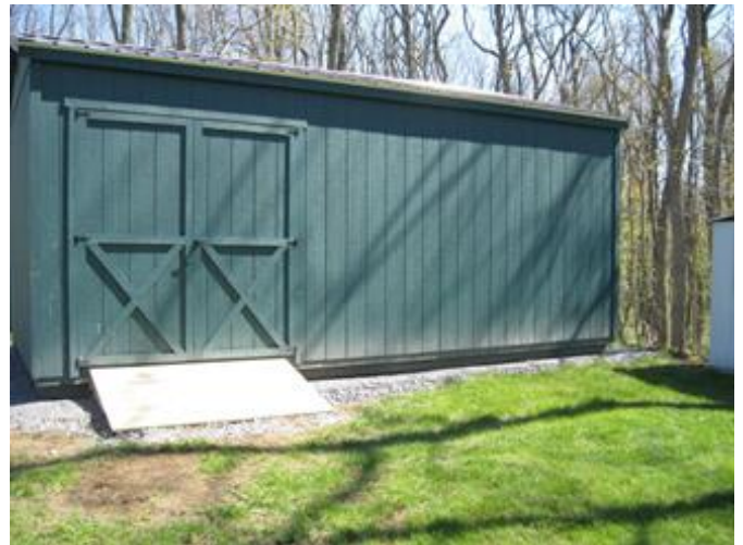
The mineral storage shed in place.
